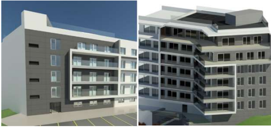
Figure 4 – Main facade with adherent tiles in porcelain stoneware, left and rear facade with fiber cement plates, right.
